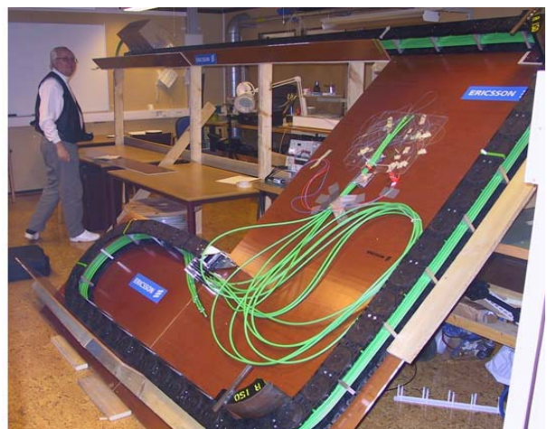
Figure 16: Testing optical cables in a chain
